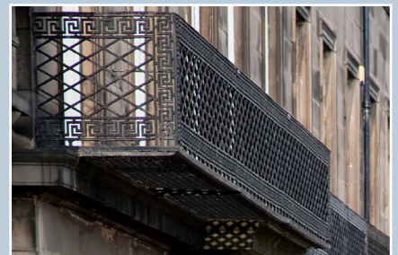
A cast-iron balcony marking the principal room on the first floor of a townhouse in Regent Terrace, Edinburgh, part of the development planned by William Henry Playfair in 1825 and built 1826–33. © N. Haynes.
