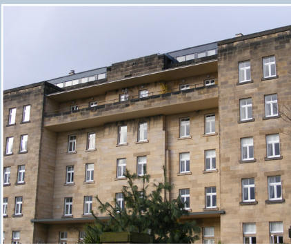
Former nurses' home of 1938–47, Salisbury Road, Edinburgh. The additional rooftop storey is set back from the wallheads, minimising its impact on the original design.
