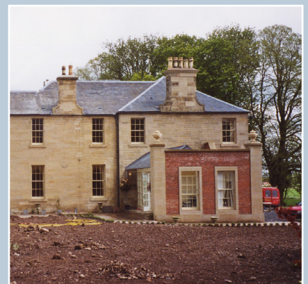
A complementary addition to a 19th-century country house in the Scottish Borders, in which brick takes its cue from walled gardens.
