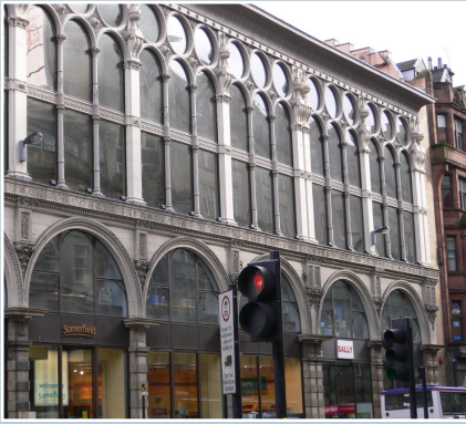
Restoration and replication: Ca D'Oro, Union Street, Glasgow. Designed by John Honeyman in 1872 in the style of a Venetian palazzo, this former furniture warehouse was extended by two replica bays (right-hand side of image) in 1989 and the roof was restored to its original profile.
