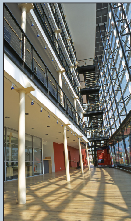
Kilncraigs Business Centre, Alloa. Above: cast-iron columns are retained internally behind the glazed curtain wall constructed in 2000. Below: A 19th-century woollen yarn store was skilfully extended in contrasting concrete and steel (left-hand side of photo) in 1938 by William Kerr. Most of the very deep original but multi-phase block (right-hand side of photo) was cut back and a new curtain wall added to the existing structure in 2000, making an assertive but revealing contrast of new and old, and achieving a visual link between Alloa Tower and the town. Junctions are clearly formed in red and white.
